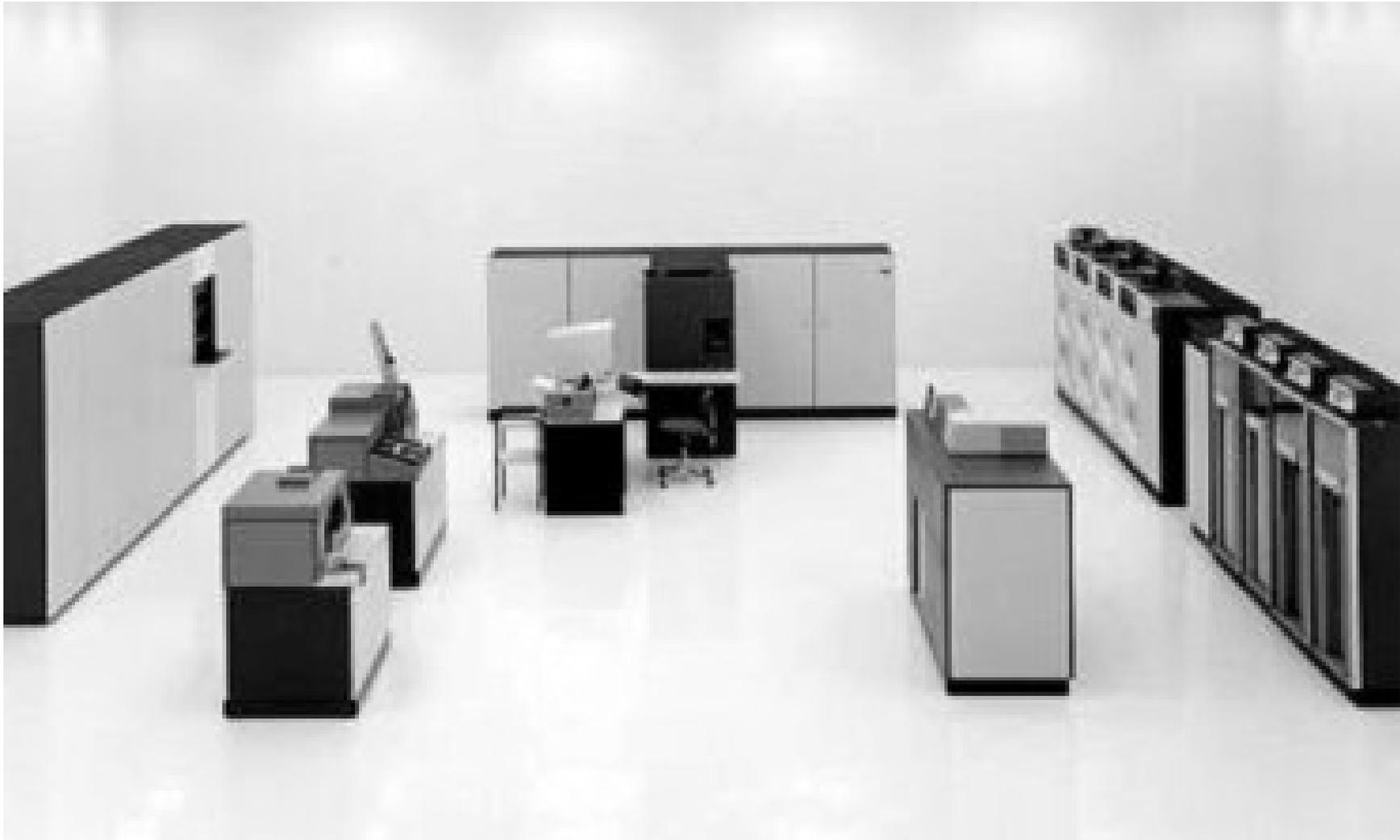
Likely devices left to right: 3850 mass storage, 3505 punch card reader, 3525 punch card reader, punch & print, processor & channel control units with operator console, 3211 printer, 3330 disks storage, 3420 magnetic tapes. From [https://www.ibm.com/ibm/history/exhibits/mainframe/mainframe\\_PP3158.html](https://www.ibm.com/ibm/history/exhibits/mainframe/mainframe_PP3158.html)
